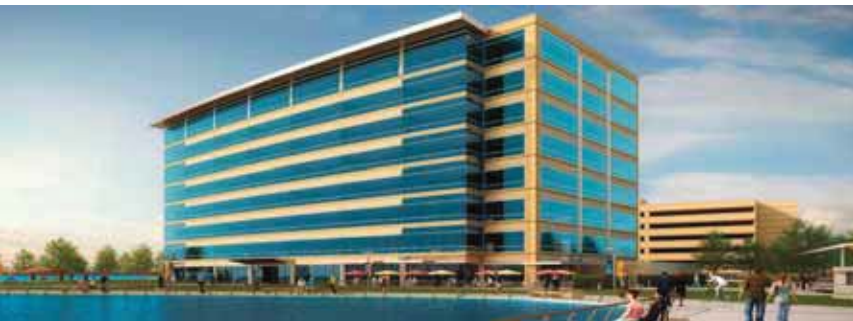
ONE HUGHES LANDING, HOUSTON, TX
